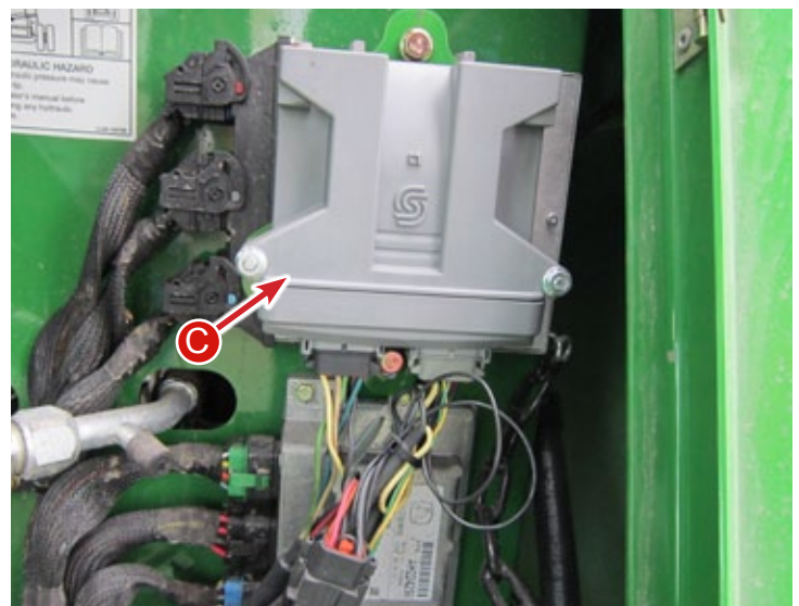
C - Leveling Controller
