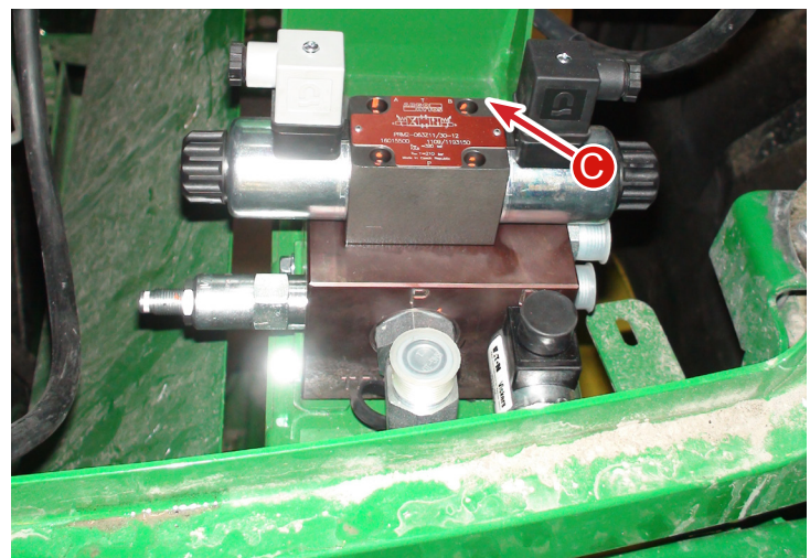
C - Leveling Manifold
